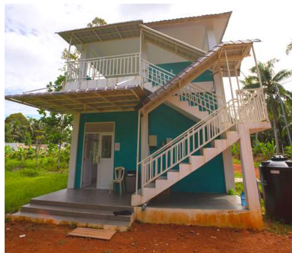
The Wak Gatak Rescue and Rehabilitation Center Clinic. Other buildings include large aviaries and a quarantine area.
