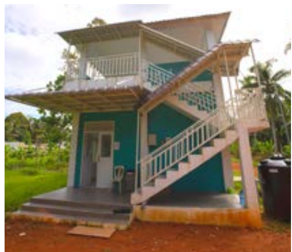
The Wak Gatak Rescue and Rehabilitation Center Clinic. Other buildings include large aviaries and a quarantine area.
